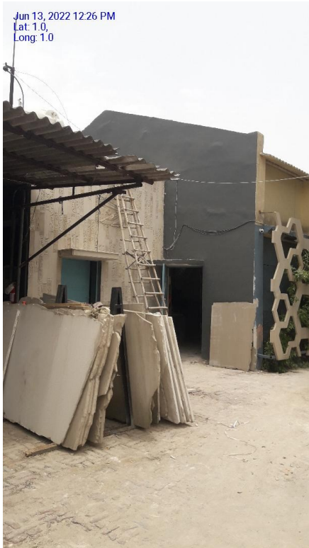
Site Exterior Picture
