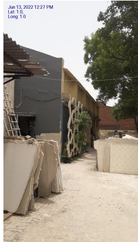
Site Exterior Picture
